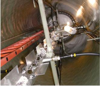
UHF Antenna mounted in self supporting GRP cylinder
