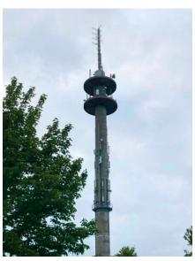
Broadcast Station "Otterndorf", Germany FM Antenna System with very low wind load
